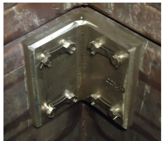
Crack damaged corner reinforced with CCRM™.
